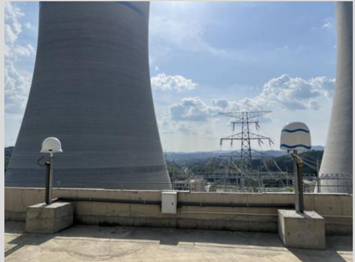
electric power plant
