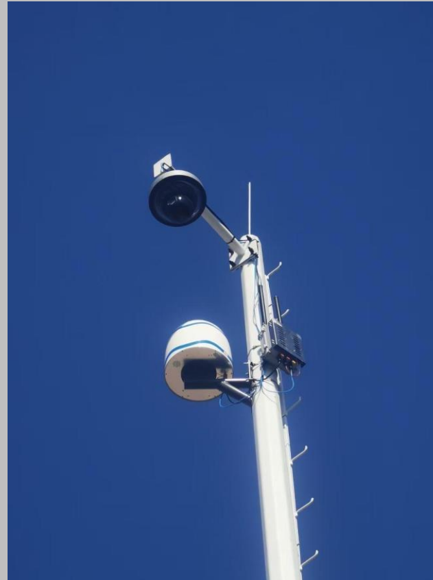
Along the High Speed Rail
